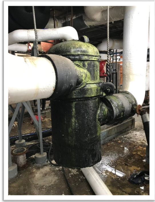
Figure 13: Expansion Tank Insulation to Replace
