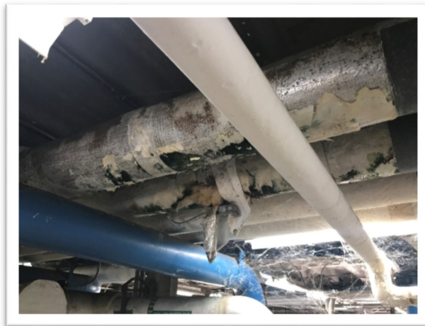
Figure 11: Damaged Pipe Insulation
