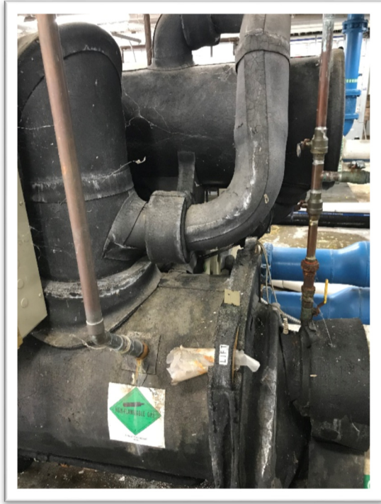
Figure 12: Chiller Insulation to Replace
